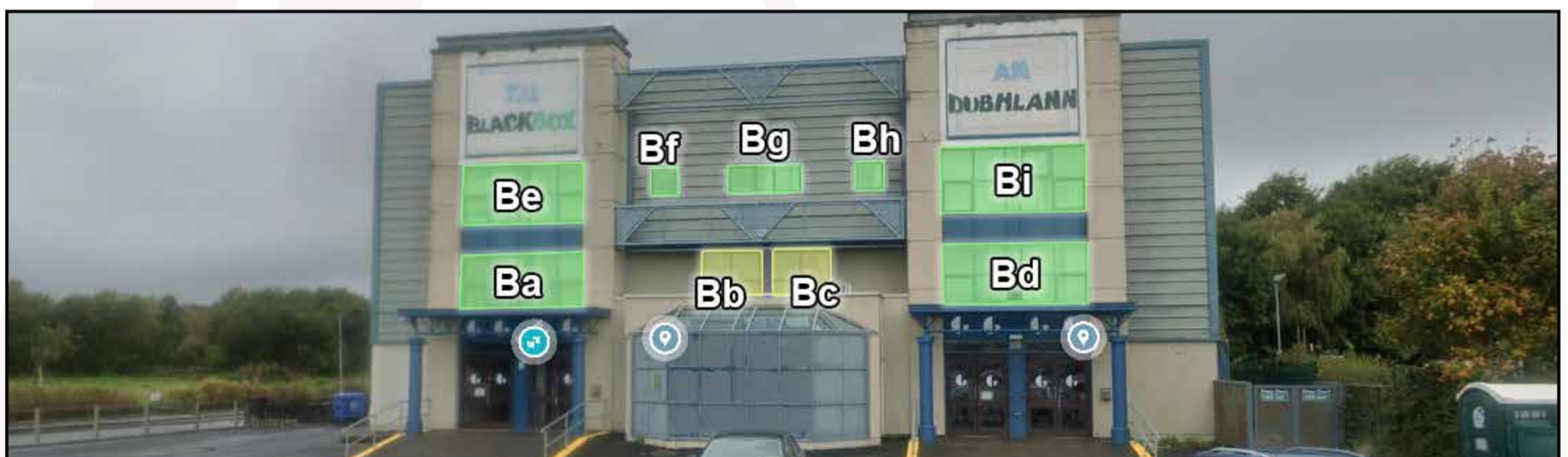
Figure 5.2: The Black Box. Windows/rooms categorised as ' negligible ' In green, ' minor adverse ' In yellow.
